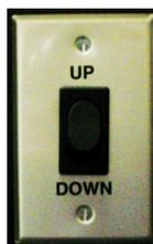
The middle position stops either upward or downward movement. The switch should be moved to the middle position after each use.
